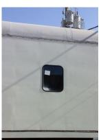
and since the Ringling years. Rubber surrounds and glass for all 22 windows were recently ordered and received, and a successful test installation has taken place. A steel door for the visitor entrance was purchased, a steel frame was constructed, and the door has been installed.
